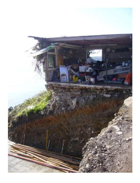
The prosecution was initiated following a routine inspection of a refurbishment project in which the building's stability had been compromised and was at serious risk of collapse. Workmen had also worked below the structure without hard hats. The contractor pleaded guilty in the Magistrates Courts and was fined £3,600.
