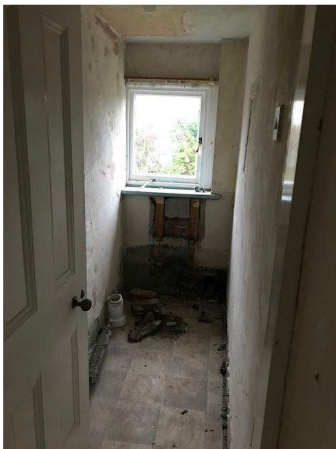
Toilet at First Floor Level
