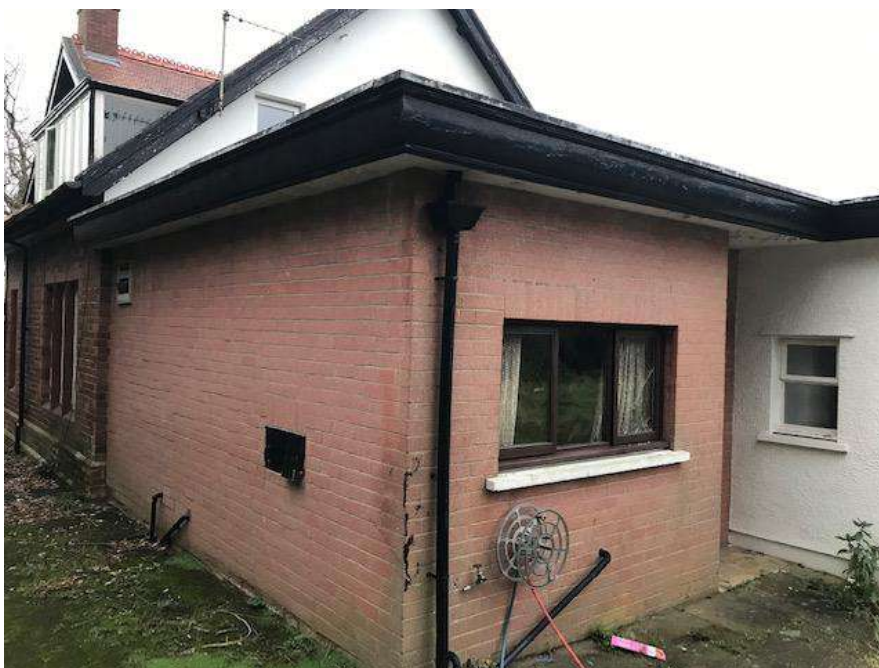
Rear and side extension to drive
