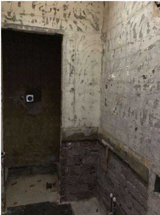
Former Shower room to extension
