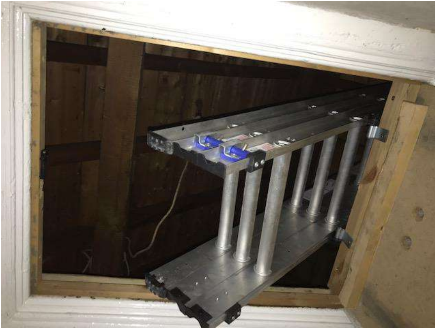
Loft hatch to landing
