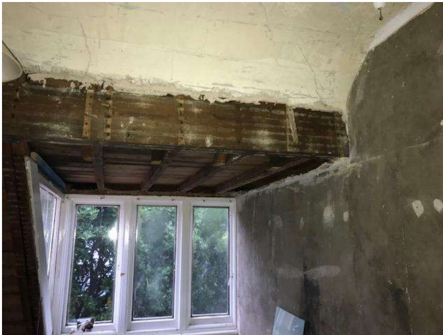
Dormer to top of stairs
