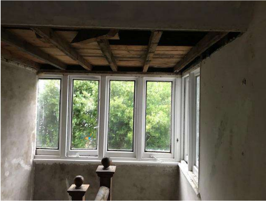
Dormer to top of stairs at First Floor
