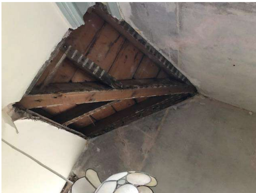
Valley boards to roof exposed in bedroom 2.
