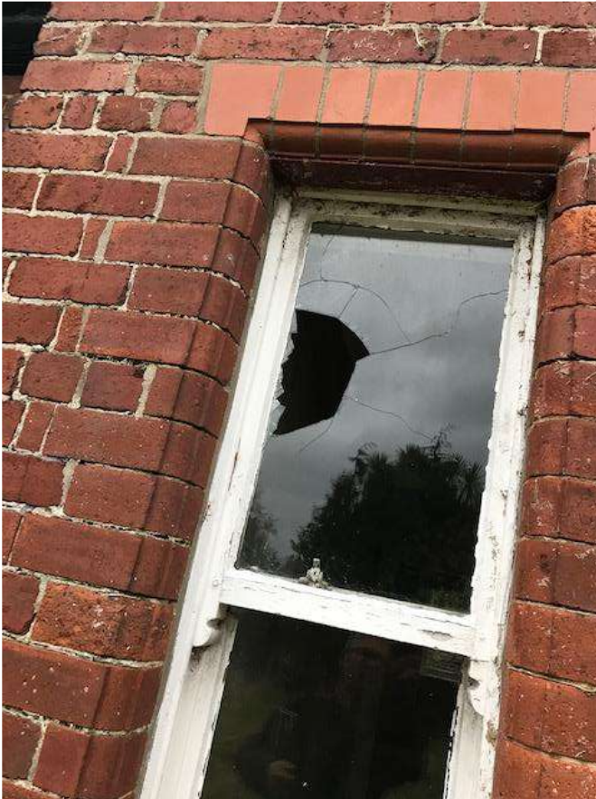
Window at ground floor to side facing garden
