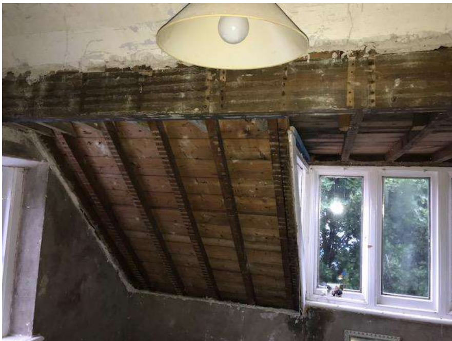
Dormer to Bedroom 3
