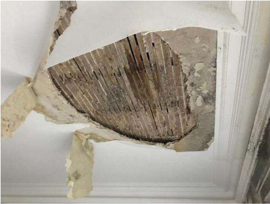
Dining room ceiling
